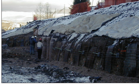
Mountain construction requires extensive shoring.
