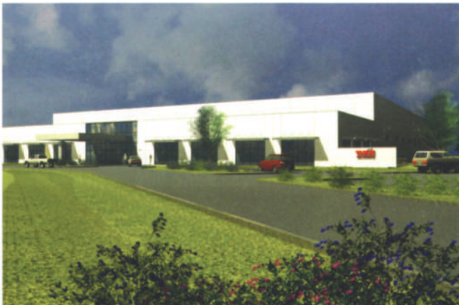
The future $7.5 million Tasus Corp. plant will sit on a 13-acre site in Georgetown and feature tilt-wall concrete slabs, a structural steel frame and, yes, a bit of feng shui.
