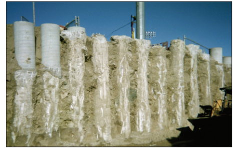
Above: Due to existing construction and underground utilities, Sky Sox Stadium in Colorado Springs is outfitted with a secant wall.
