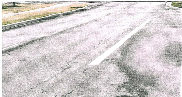
Frisco, Texas, engineers thought excessive amounts of the mineral ettringite in the city's soil was distressing roads and streets. After retaining a consulting firm to test the soil, however, they learned that the culprit is clay, which soaks up water and can expand up to 15 times its original size. Photo: CTL | Thompson Inc.
