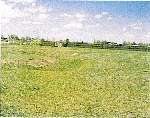
Sugar beet waste can create caves and sink holes that impact soil stability, causing foundation movement and differential settlement of buildings.
